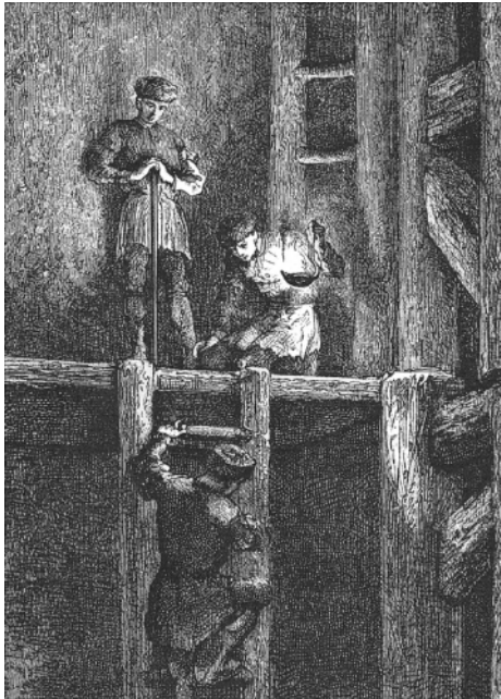
The spacious ladder shaft in the Harz mines, N. Germany. Simonin.
