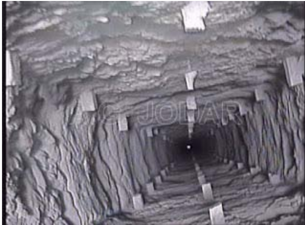
The extraction shaft of La Guzman, the guide rail fittings can be seen.
