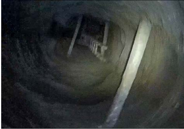
Looking up the ladder shaft.
