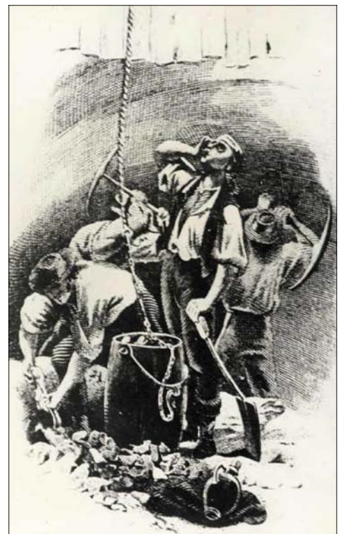
'Mucking off' or clearing the debris.
