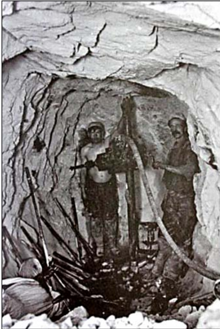
Single line pneumatic drill, known as a widow maker.
