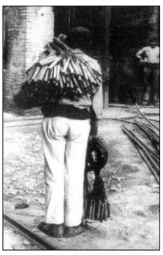
The menchero carried the fuse cartridges to the barrenos.
