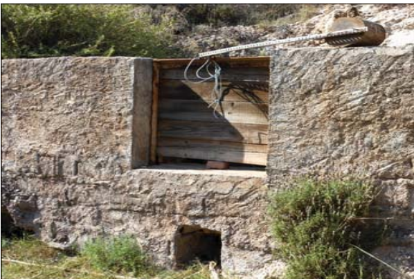
The sluice gate and the entrance to the water channel under the hill.
