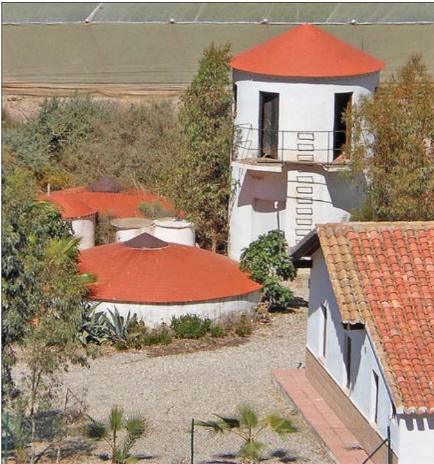
“Rapunzel's Tower”, the water filtration and storage system next to the doctor's old house.
