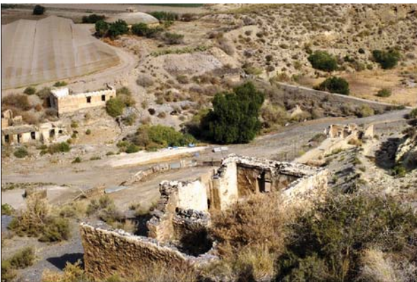
The wall damming the Rambla del Arteal can be seen in the centre right of the picture.
