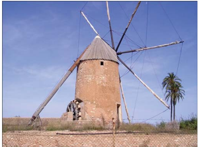
Remains of a wind powered noria. Spanish Waterworks. Jill Dickin Schinas.
