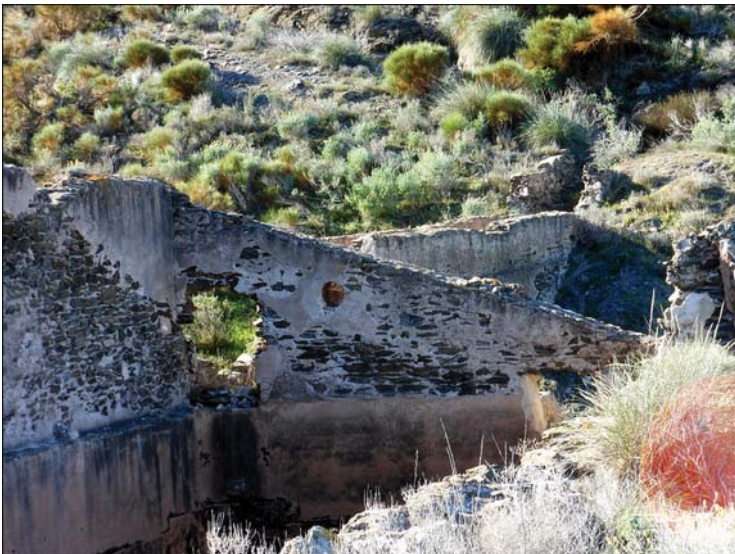
Water from one slope entered the balsa at this end via the aqueduct.
