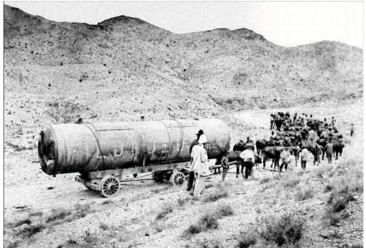
The boiler for the desagüe arrived in Villaricos in 1851 and was transported by a team of oxen. Sierra Almagrera y Herrerías. Bolea.
