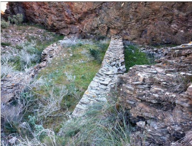
Above, the low wall used to conduct the water.
