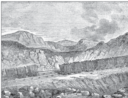
Empty and full trucks on a simple inclined plane.
