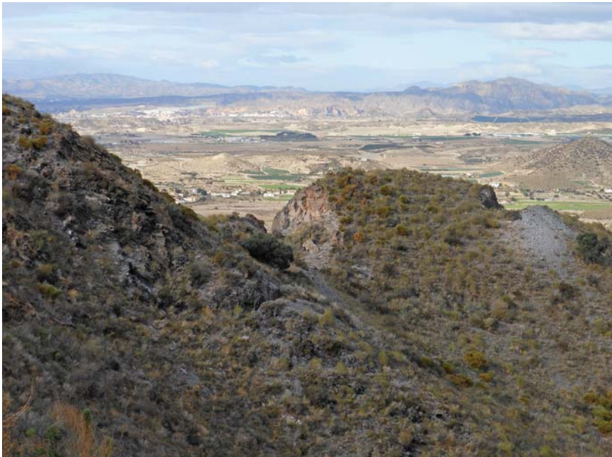
The cutting on the right was made for the Los Tres Pacos cable, the one on the left was for the railway line from Centinela.
