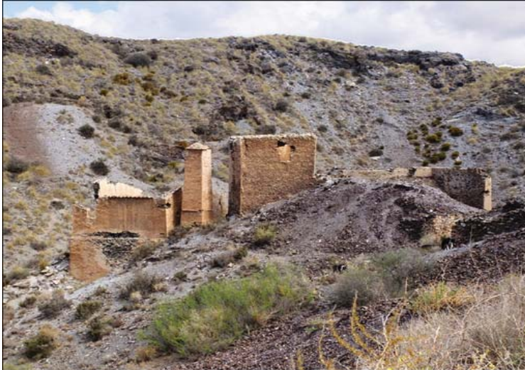
The remains of the Violeta loading station at República Romana.
