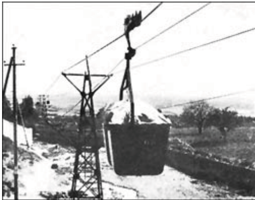
A tri-cable system similar to the type used on Los Tres Pacos line. Adurcal.com
