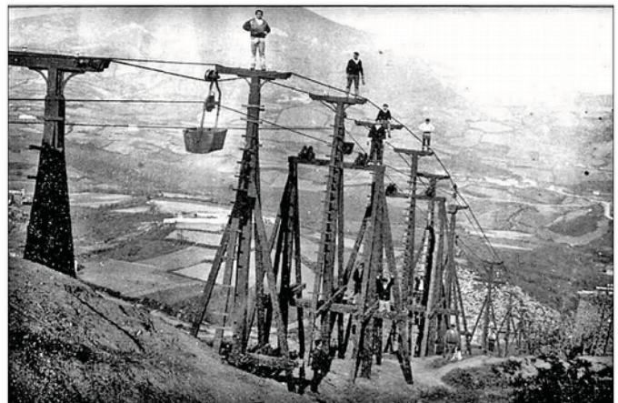
An aero cable maintenance team.
