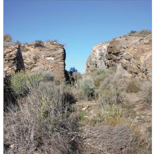
The cutting made for the buckets to clear the summit
