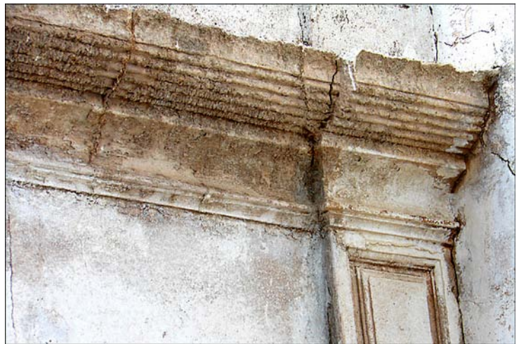
Detail of the moulding inside the chapel.
