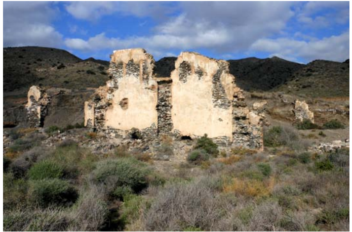
The wall seen from the other side.
