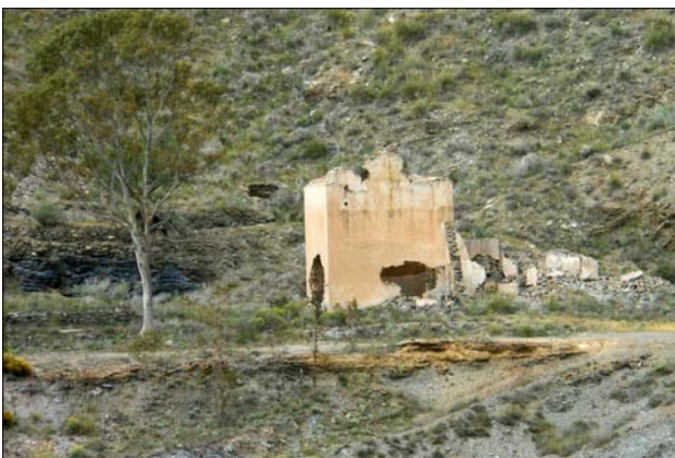
Above, Guzman's transformer.
