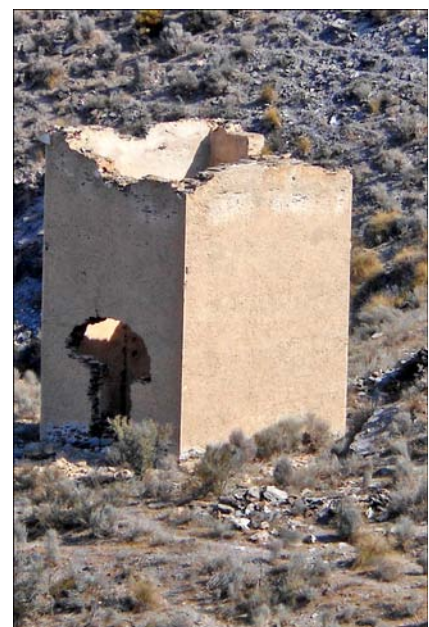
Right, Republica's transformer.
