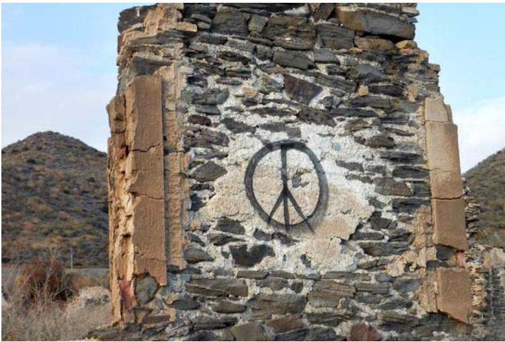
6 The generators. The generators were housed in the area between the facade and the turbines. The full facade can be seen in the 1912 photograph on page 49. This is part of what remains of it today.
