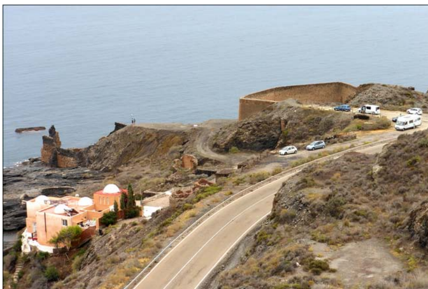
View of lower hopper, cargadero and calcination ovens.
