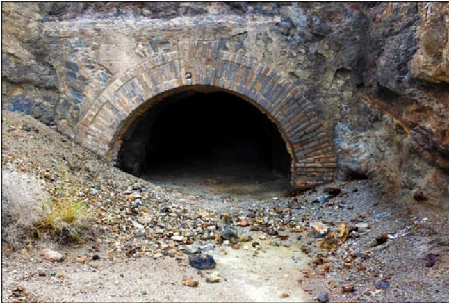
San Agustín tunnel entrance.
