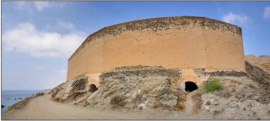
General view of lower hopper from below.
