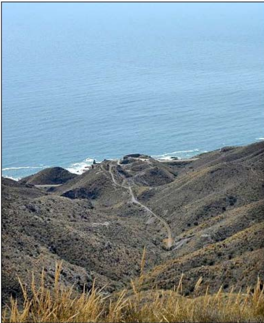
The inclined plane seen from the top of the Sierra. The lower railway line can be seen running from the plane and looping round the top of the hopper.
