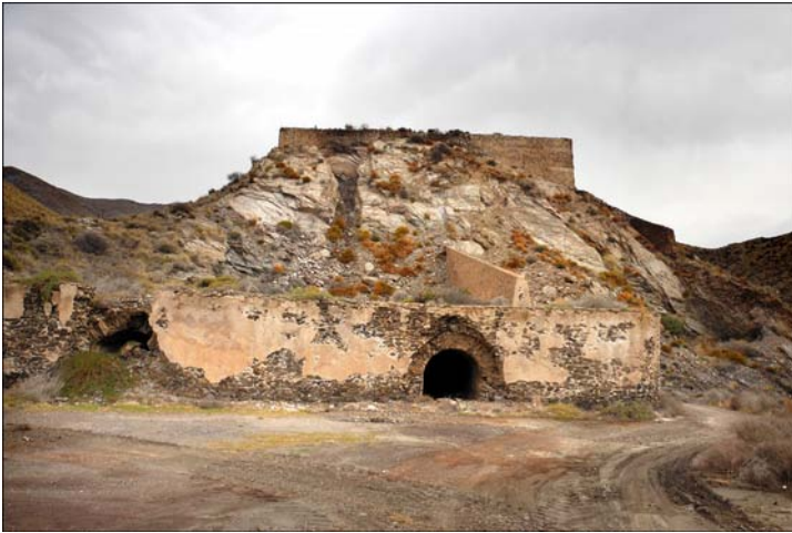
The upper hopper. The wagons tipped from the top of the wall.
