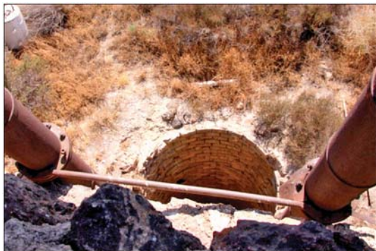
The Ana Josefa shaft, where the pumps were housed, is situated under the structure to the left of the chimney.
