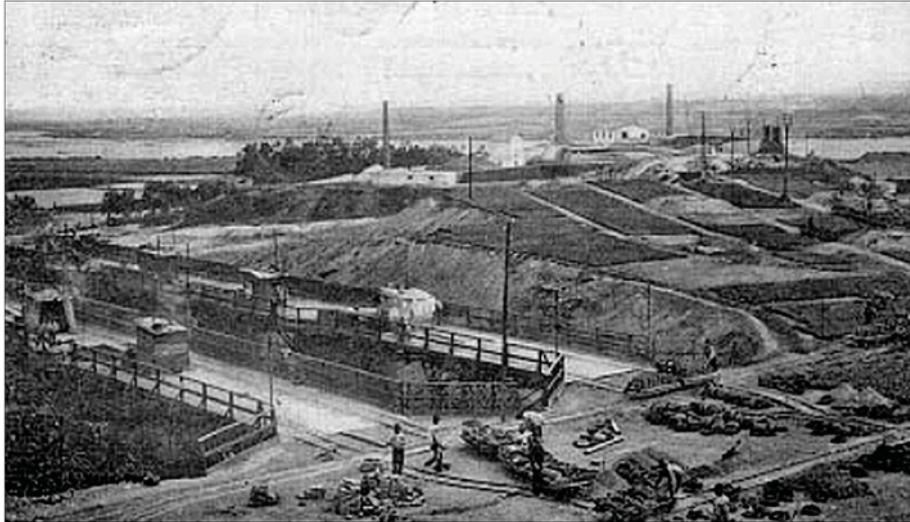
The contention wall, seen on the right-hand side of the picture, was vital in keeping the Rozas dry. E.L.Morin
