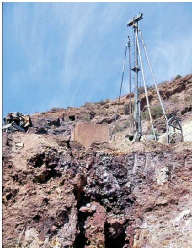
Probing for old workings using a percussive drilling rig.
