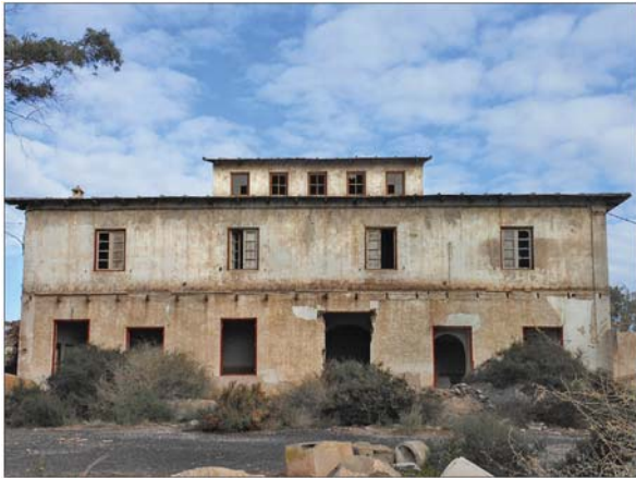
The engineers' accommodation.
