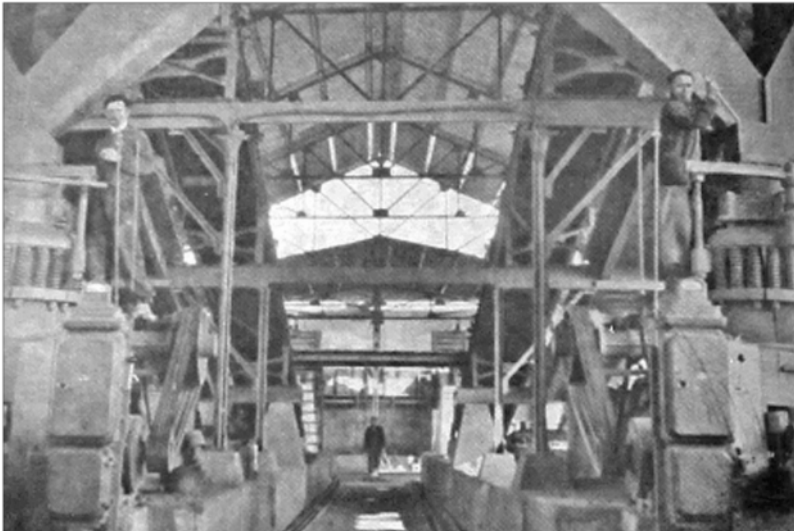
Inside the shorter of the two sheds. Minas de Almagrera S. A. Sánchez Picón
